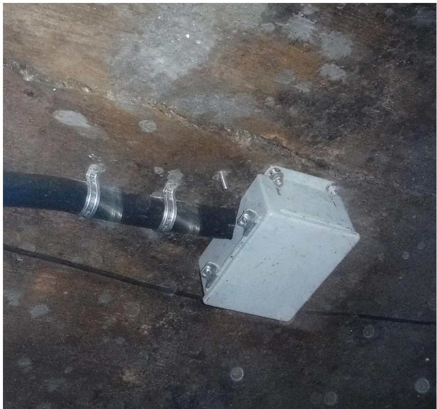
Figure 2. A geophone installed in a wastewater tunnel.
